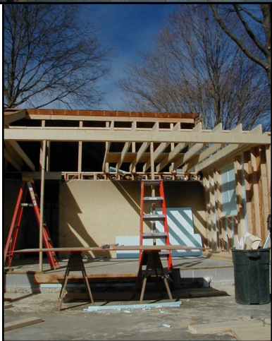
New roof system installation
