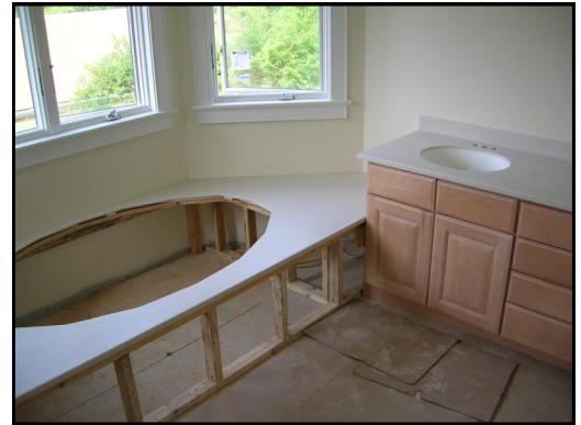
Master bathroom tub deck
