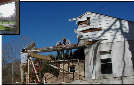
Removal of existing roof system
