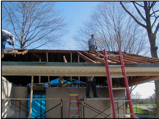
Removal of existing roof system
