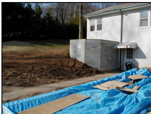
Master bathroom block foundation
